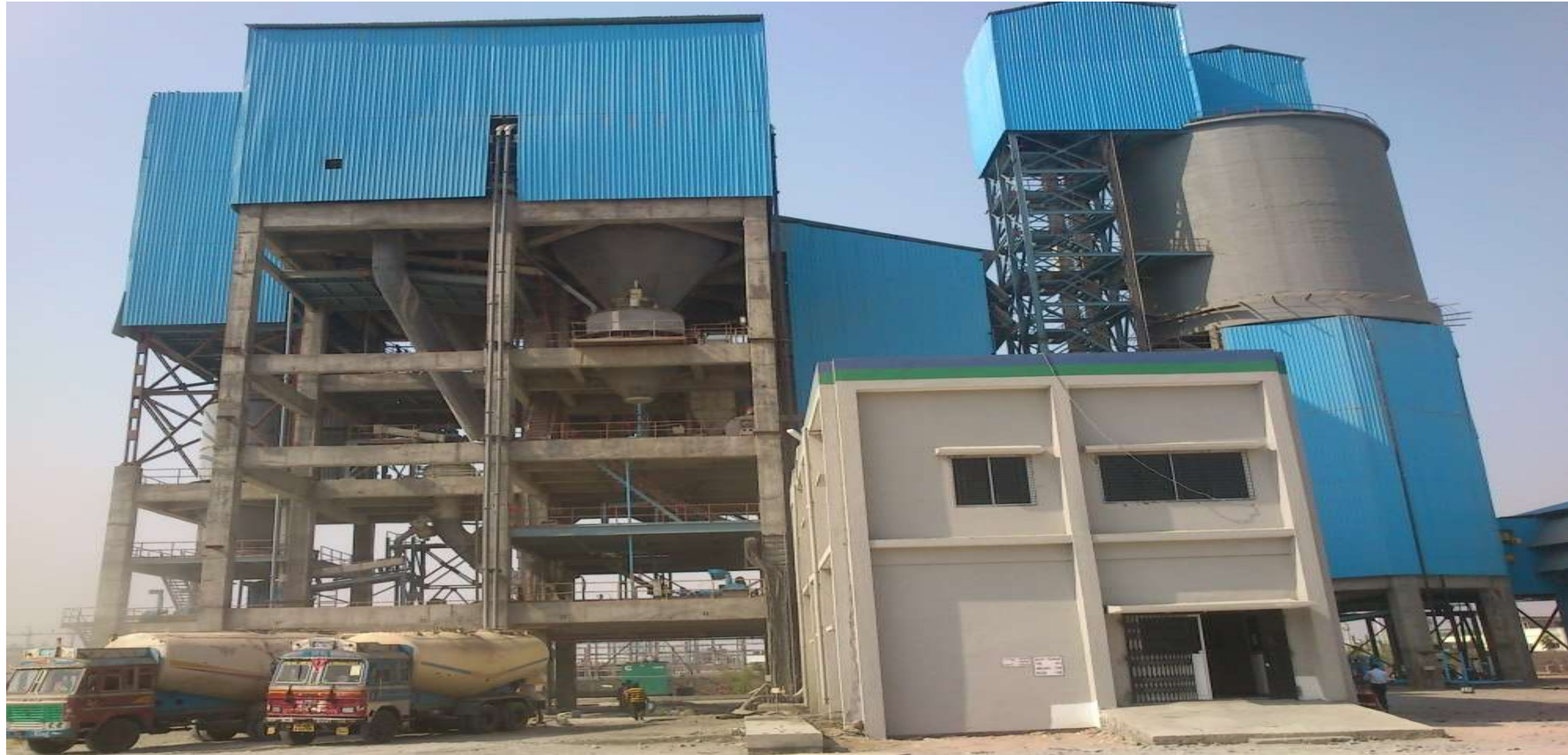
Cement blending & packing plant 1500 TPD @ Raichur
