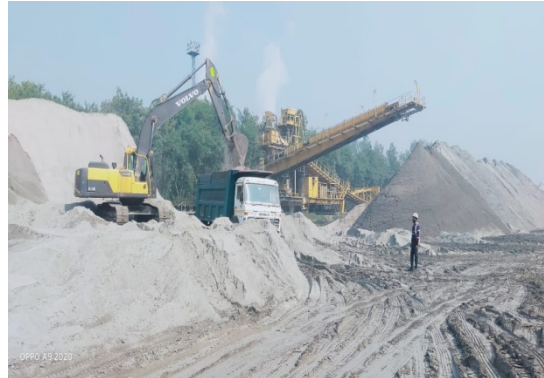
Loading from Open Yard
