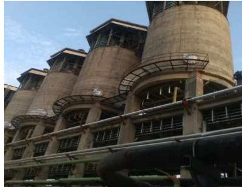
6000 MT Dry fly ash Silo installed
